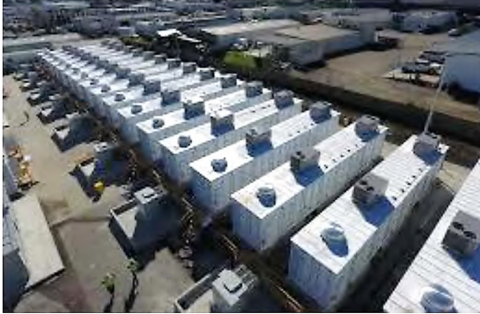
Photo PD-3: Examples of Battery Storage Containers
