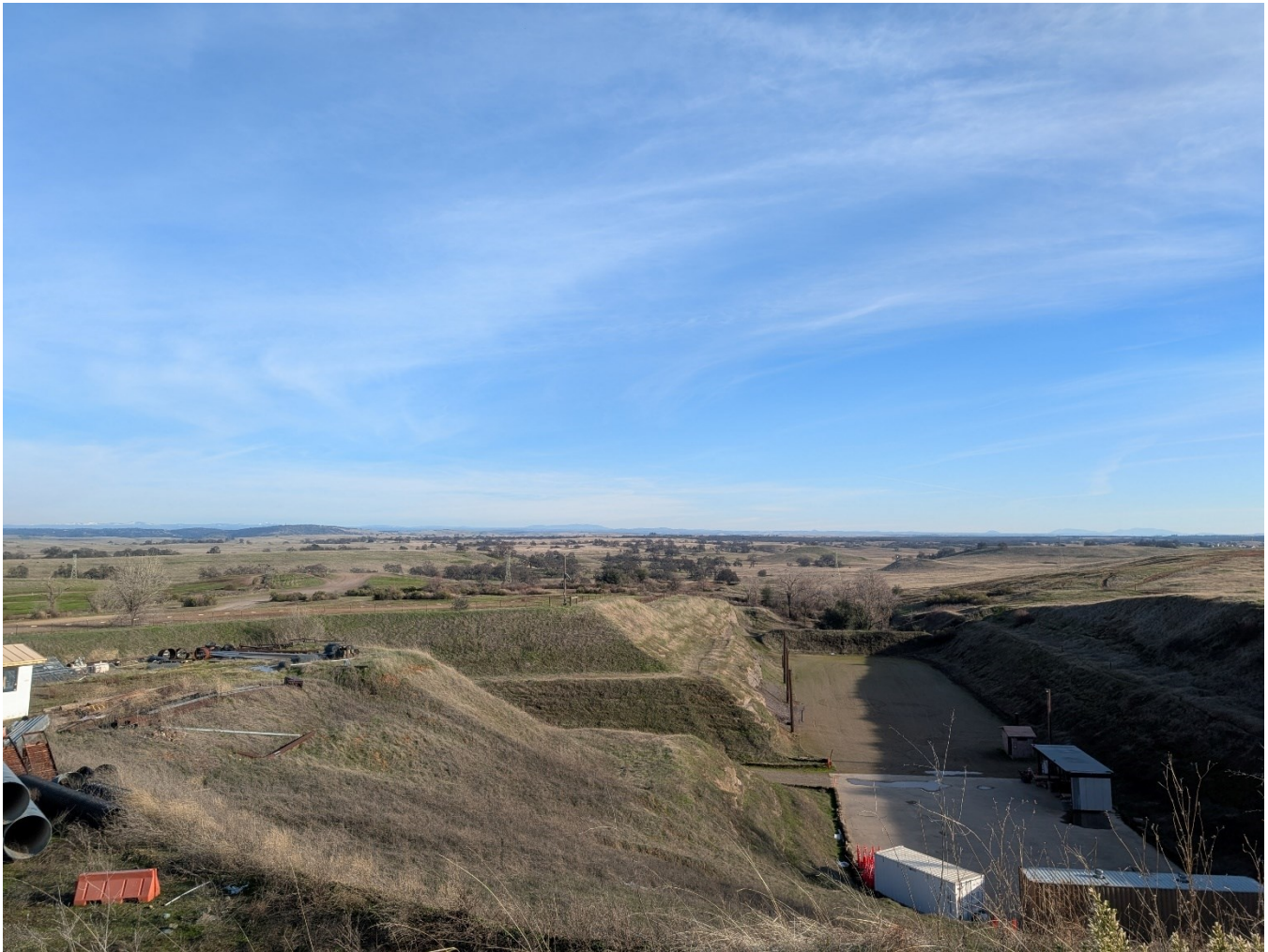
KOP 9h. Looking Southeast from the Prairie City SVRA Picnic Area/Overlook. Construction equipment and improvements associated with the former shooting range in the foreground; oak woodlands, trees, rolling grassland and utility poles in the middleground; and trees, foothills, and the Sierra Nevada visible in the background.
