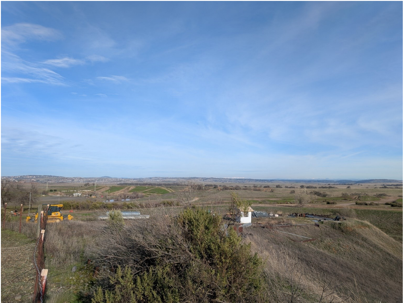
KOP 9f. Looking East/Northeast from the Prairie City SVRA Picnic Area/Overlook. Grassland, shrubs, and a wire fence are visible in the foreground. A construction staging yard containing heavy construction equipment, metal piping, and other miscellaneous objects is visible in the background. Additional grasslands, scattered trees, buildings, and the rolling hills of the Sierra Nevada are visible in the background.
