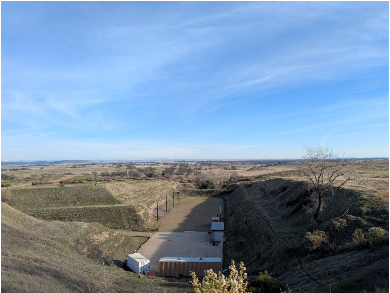
KOP 9c. Looking Southeast from the Prairie City SVRA Picnic Area/Overlook east of the Environmental Training Center. Trailers, power poles, concrete, and other improvements associated with the former shooting range are in the foreground. Oak woodlands and rolling grassland is in the middleground and the Sierra Nevada foothills and Sierra Nevada are visible in the background.
