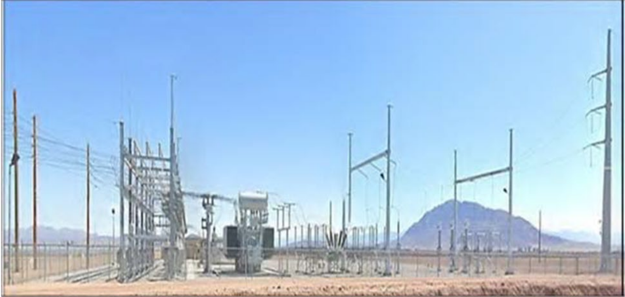
Photo PD-2: Proposed Project Conceptual 230 kV Substation.
