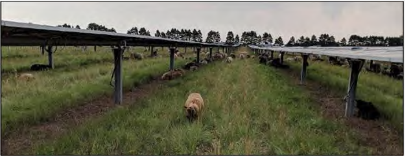
Exhibit 2D. Sheep grazing and resting amidst solar panels for vegetation management on another project.
