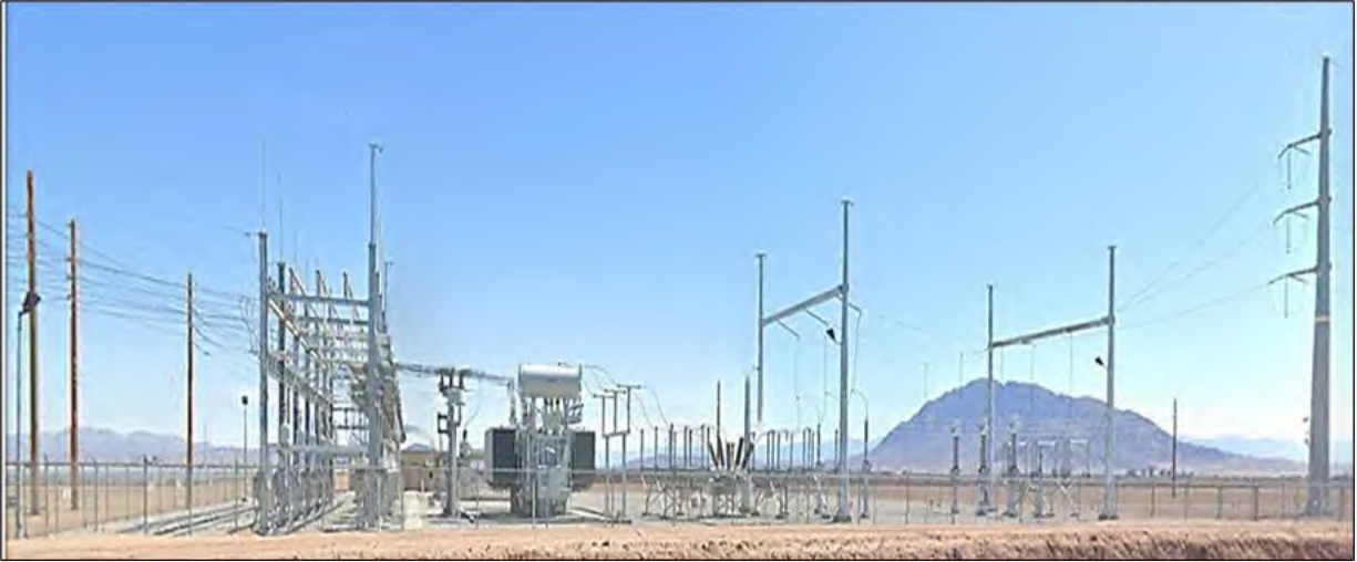
Exhibit 1C. Proposed project conceptual 230 kV substation.
