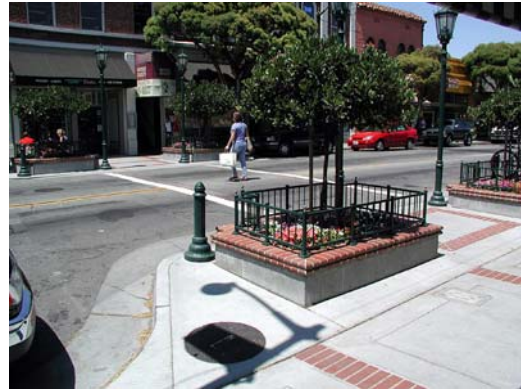
Figure 14 Mid block crossing on internal streets
