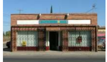
This existing building on M Street displays the site design desired for buildings on M, Front, and West Front Streets with the building constructed to the back of the sidewalk at the front of the property. (The security grill is not recommended as a design feature).
