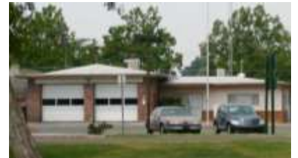
Rio Linda Fire Station showing original brickwork
