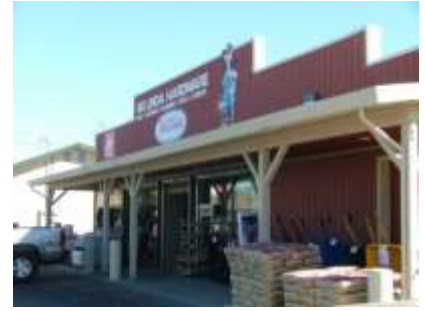
A typical commercial building, with flat roof and false front, wood siding, and an awning
