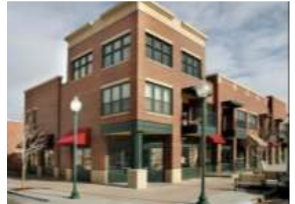
The third story incorporated into the corner of this mixed-use building allows for additional square footage without compromising the building's human scale. Varied setbacks and rooflines provide visual texture and articulation.
