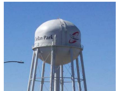
The McClellan Park water tower with the painted logo is an example of an oversized Business Park sign
