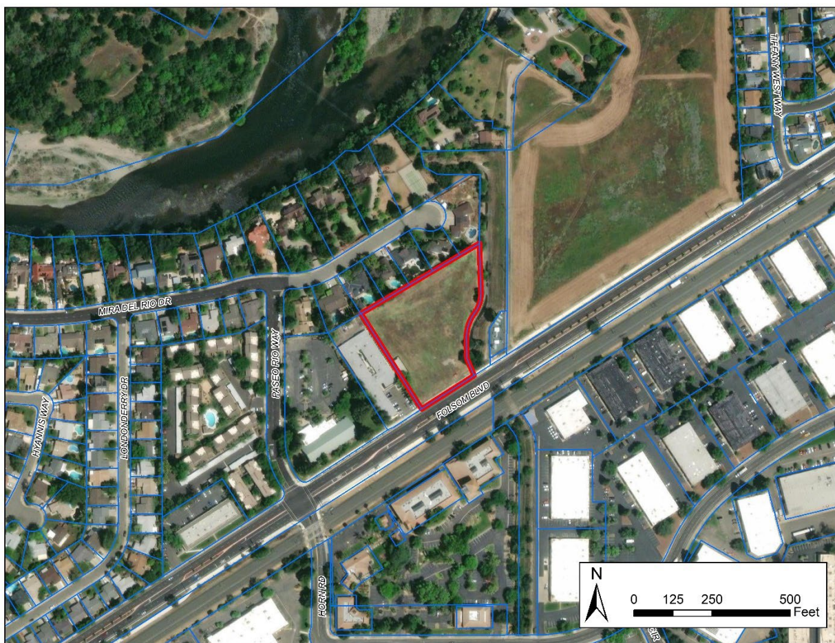
Figure E-11: Site 16
