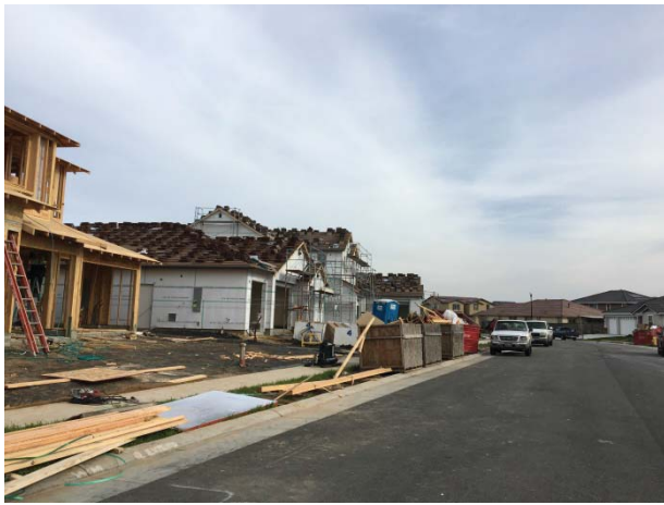
Homes under construction
