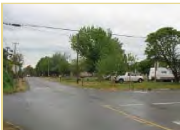
Existing conditions at the intersection of I and 34th Streets are typical of the Corridor Plan Area of Influence
