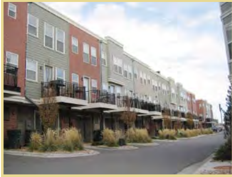
Tuck-under parking for these residences is accessed through an internal alley.
