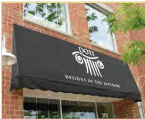
Awning colors should be selected to contrast with the sign message and should be compatible with the color and materials of the wall surface.
