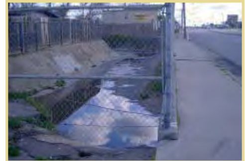
Magpie Creek and creeks and drainage-ways on the east side of the Corridor Plan area have been channelized and may be enhanced to serve as urban greenways.
