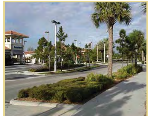
New east-west local streets will be needed to serve infill development in the Corridor Plan area.
