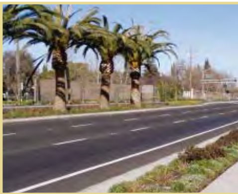
Streetscape improvements on Watt Avenue (shown between Peacekeeper Way and Palm Avenue) will be constructed progressively northward.
