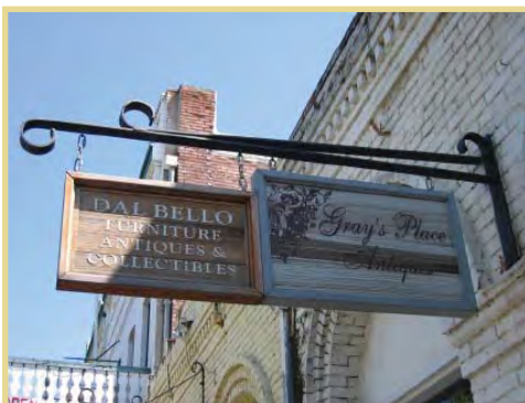
Pedestrian signs are suspended from a support that projects perpendicular to the wall surface.
