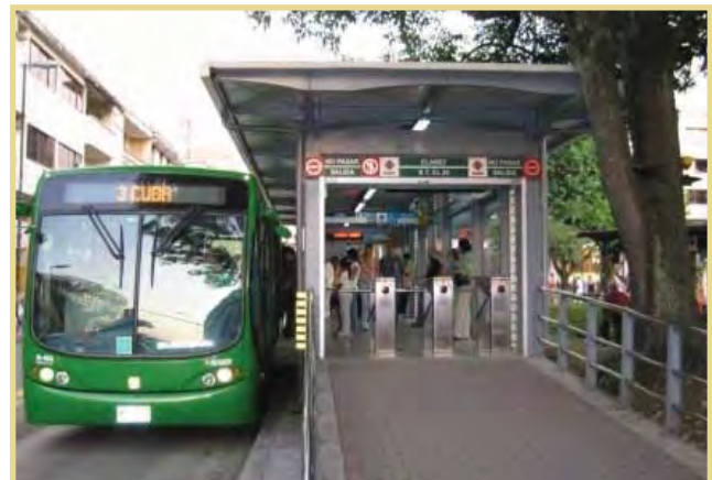
Bus rapid transit facilities will include pay stations to facilitate fast and efficient operation.
