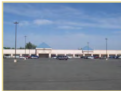
The County's North Neighborhood Services Center is located in one of the existing commercial/retail centers in the North Highlands Town Center.
