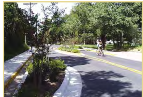
Chicanes are curb extensions that alternate from one side of the street to the other to create S-shaped curves.
