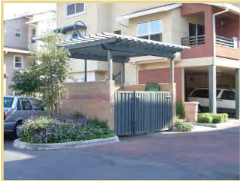
Trash enclosures should be screened to blend in with the surrounding site architecture.
