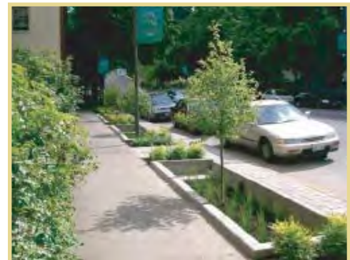
Planter boxes collect stormwater runoff, helping to irrigate landscaping.
