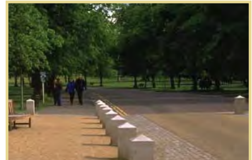
Bollards should be used to restrict vehicular access where trails intersect streets.
