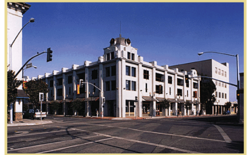
Watt Avenue will be a commercial street with defined districts and community destinations.
