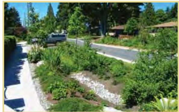
Drainage swales along this neighborhood street filter runoff from the street and sidewalk.
