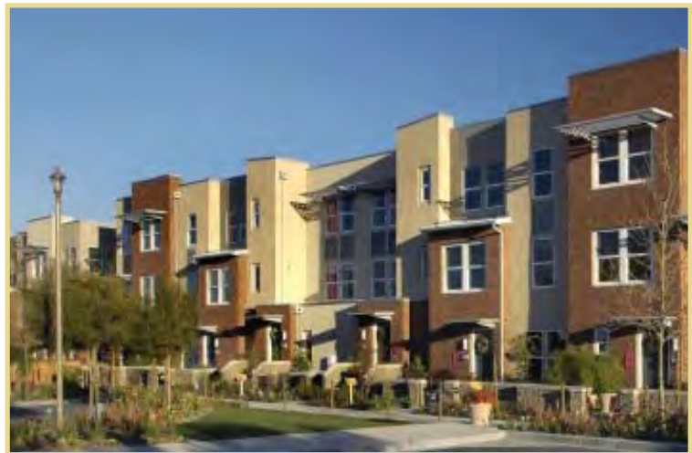
Housing densities in the Elkhorn District Center should be sufficient to support bus rapid transit.
