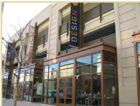
Parking structures should be designed with architectural features that integrate them into the community.
