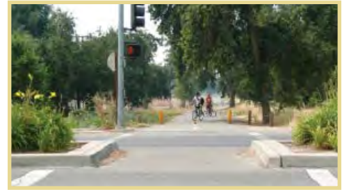
Traffic signals should be installed to enhance the safety of trails across major streets.
