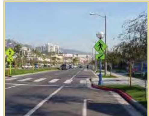
"Complete streets" can include sidewalks, planting strips, bicycle lanes, and enhanced pedestrian crossings to improve street function and the experience for pedestrians and cyclists.
