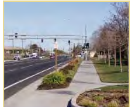
Streetscape improvements on Watt Avenue will be extended to Antelope Road.
