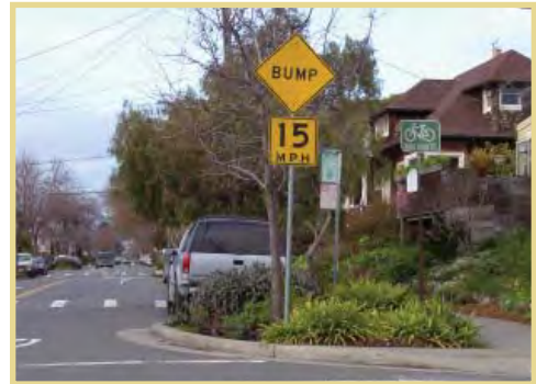
Bulb-outs at intersections reduce the crossing distance.
