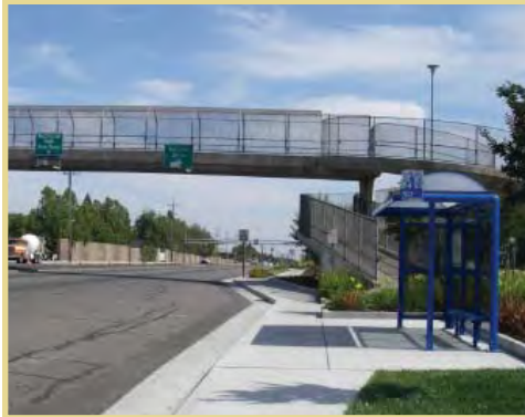
Streetscape improvements and new local bus transit stop on Watt Avenue
