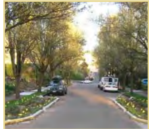
Vegetated curb extensions are used in this neighborhood green street.
