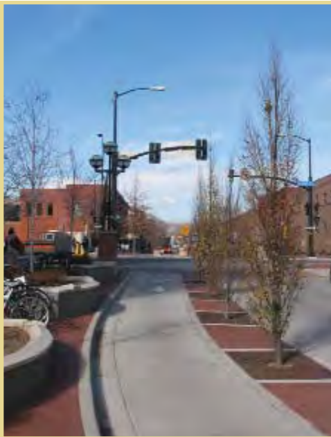
New and upgraded streets should accommodate mobility options. The street shown above provides bicycle lanes separated from the street by a landscaped strip.
