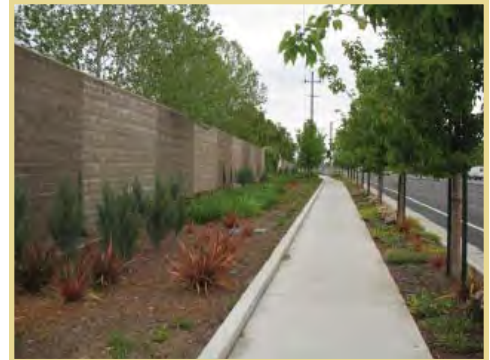
Implementation of streetscape improvements are underway along North Watt Avenue.
