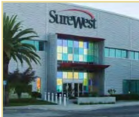
Corporate office at McClellan Business Park
