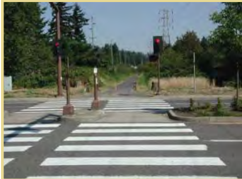
Ensure safe and convenient access at trail crossings.
