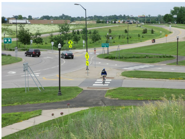
Example of a multi-lane roundabout.
