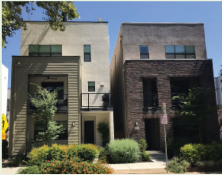
Wood, metal & brick siding
