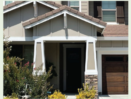
Broad tapered wood columns
