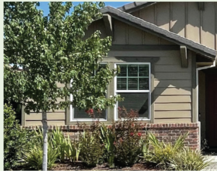
Double-hung windows with multi-plane glass
