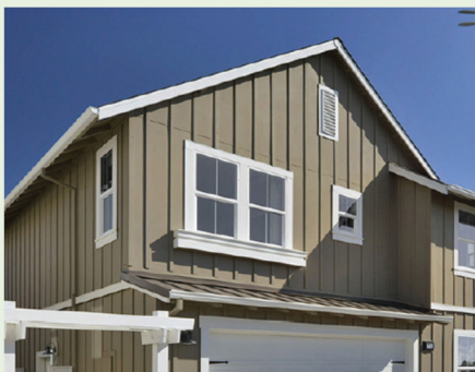
Board & batten siding
