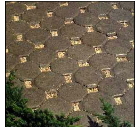
Permeable interlocking concrete pavement combines stormwater infiltration, retention, and surface use (e.g. driveway) into one place, thereby reducing runoff volume.
