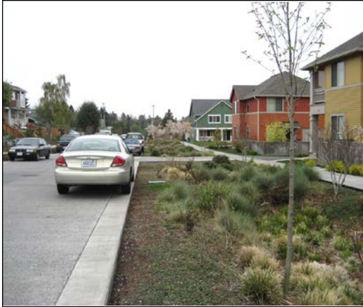
Planter strip along a local residential road is planted with native vegetation and utilized as a stormwater treatment device
